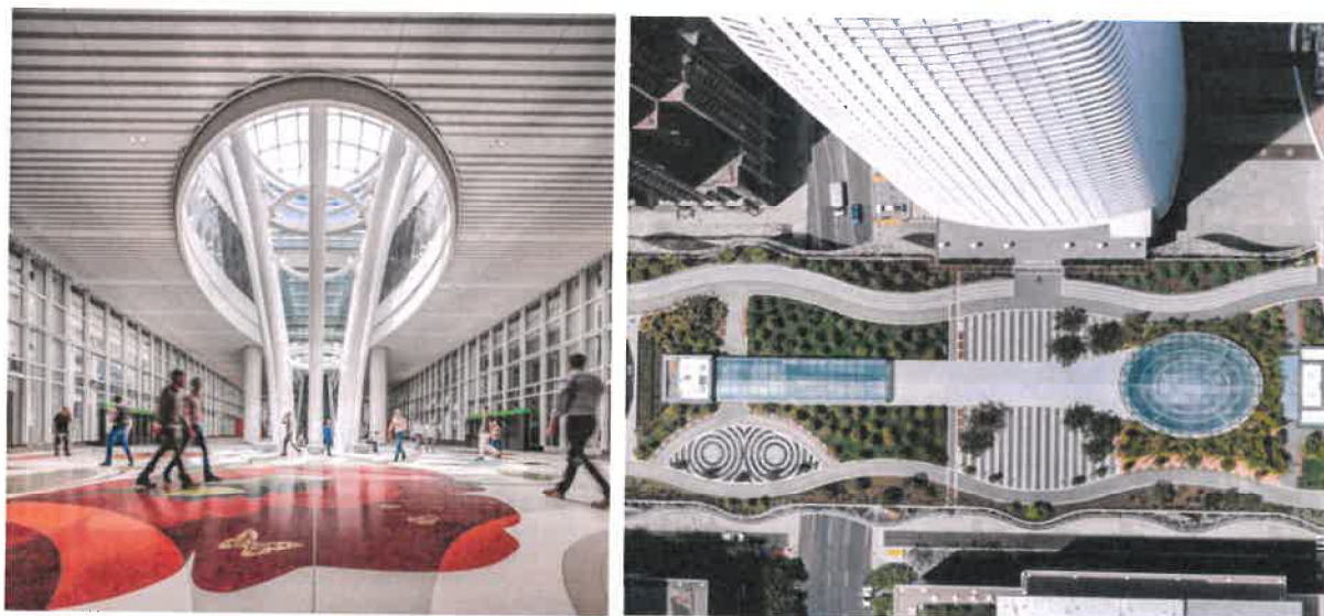
Salesforce Transit Center realizat de arhitecți Pelli Clarke & Partners, San Francisco, California USA
